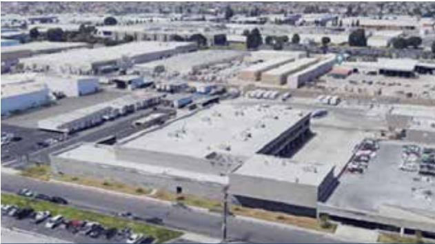
Managed the replacement of seven heating and ventilation (HV) units at the Anaheim Bus Base Maintenance Building.
