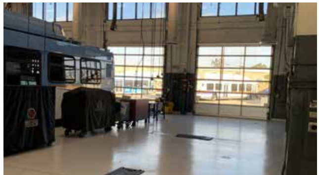
Oversaw the replacement of the maintenance building shop floors at the Garden Grove Bus Base while maintaining operations.
