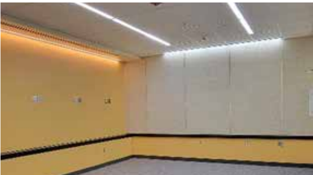
Managed the facility modification project for the I-405 Toll Operation Center at the Santa Ana Bus Base.
